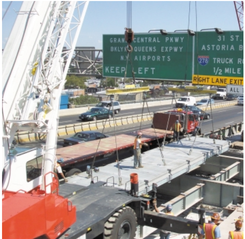
Right: Deck replacement on New York City's Triborough Bridge main span.
